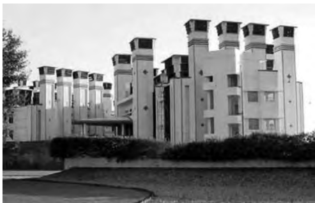
Figure-3: Passive Downdraught Evaporative Cooling in Torrent Research Centre, Ahmedabad.
