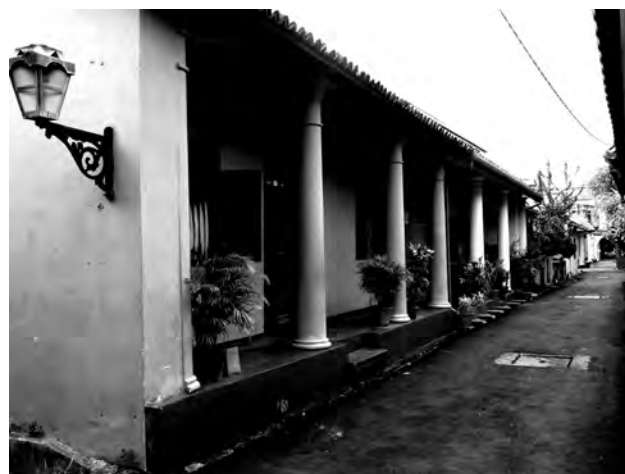
Figure-17: Restored street elevation of No. 03, Parawa Street. Source: Author
