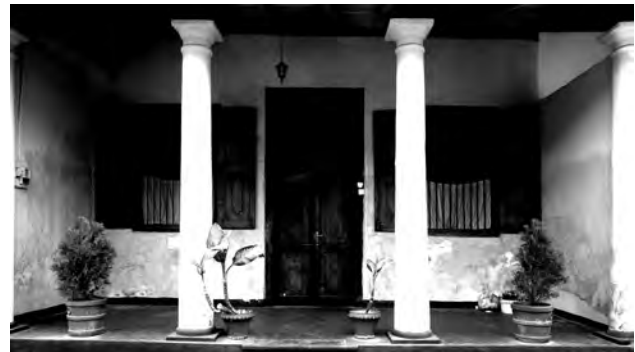
Figure-7: Restored column fronted verandah of No. 52, Leyn Baan Street. Source: Author
