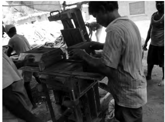
Figure-7: CSEB manual block making machine. Source: Self documentation, Auroville.
